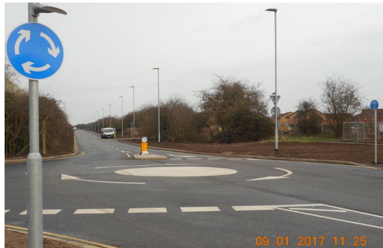
New access road at Lynnsport opened January 2017
